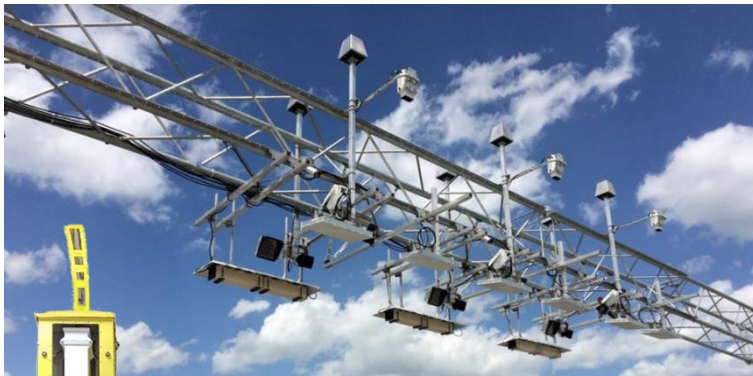
Gantry mounted PERMs (above), Radiation Portal Monitor with PERMs (left) and stand-alone PERMs in ocean port environment (right)
